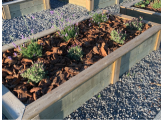
Planter boxes were installed by our maintenance team and planted by \frac{3}{4} students as part of our beautification efforts.
